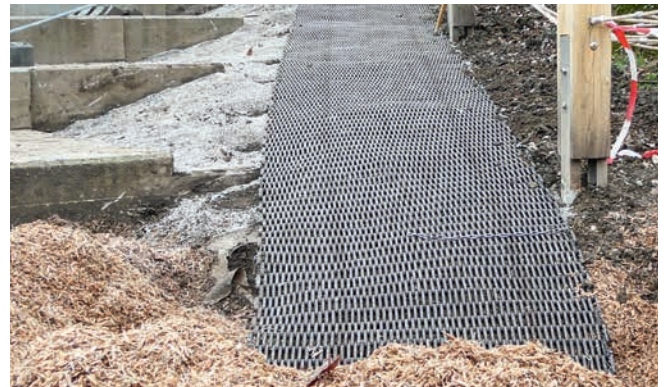
Mat directly after placing
