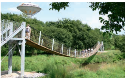
Wooden walkway bridge, Length 54 m
