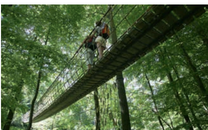
Wooden walkway bridge, Length 40 m
