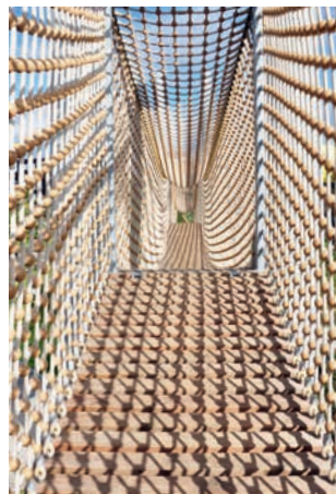
Net tunnel, square, underfoot material made from larch wooden rungs
